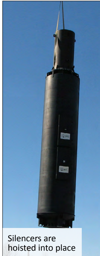
Preparing to install the silencers
